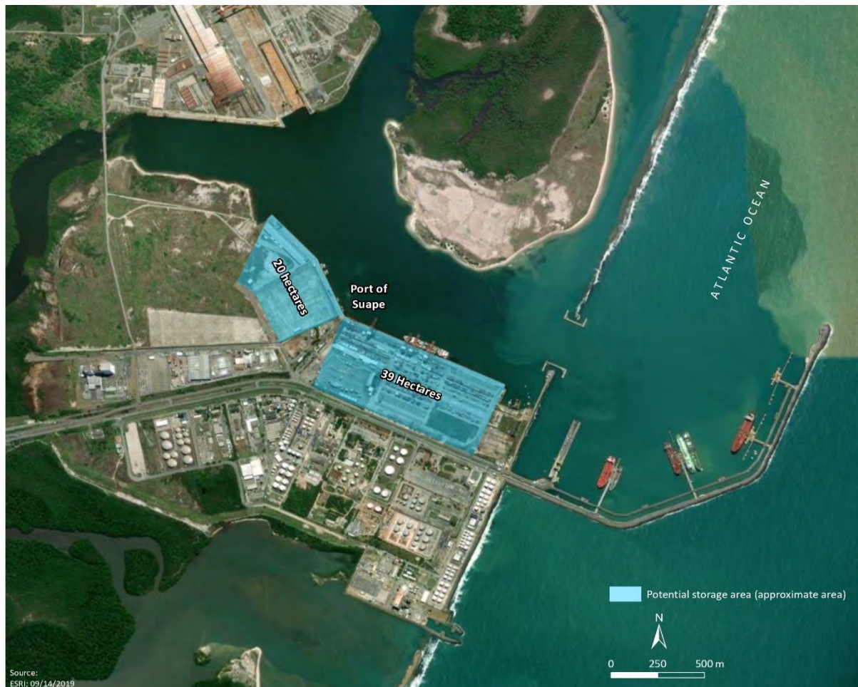
Figure 6-6: Aerial view - Port of Suape
