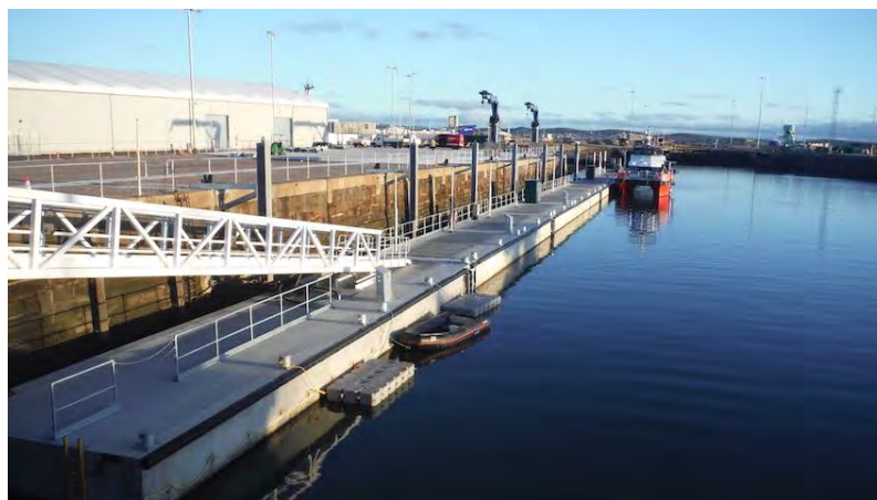
Figure 6-19: Barrow harbor with crew transfer vessel pontoon [66]
