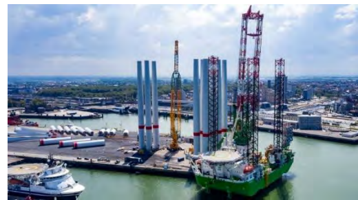
Figure 6-17: WTG pre-assembly at quayside [65]
