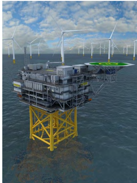
Figure 4-13: Offshore substation rendering of topside and jacket [73]
