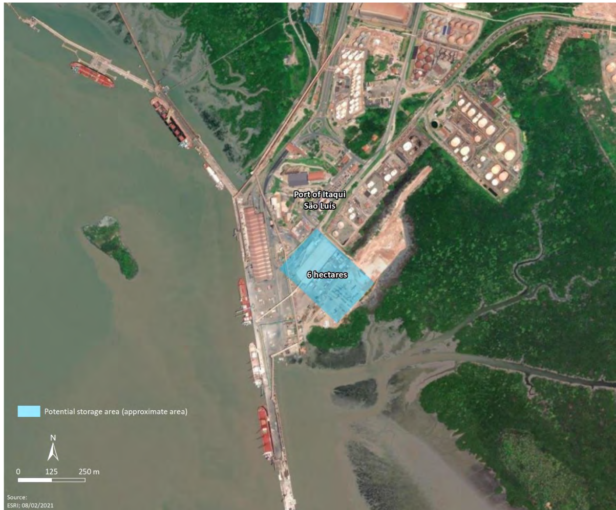
Figure 6-2: Aerial view - Port of Itaqui / São Luís
