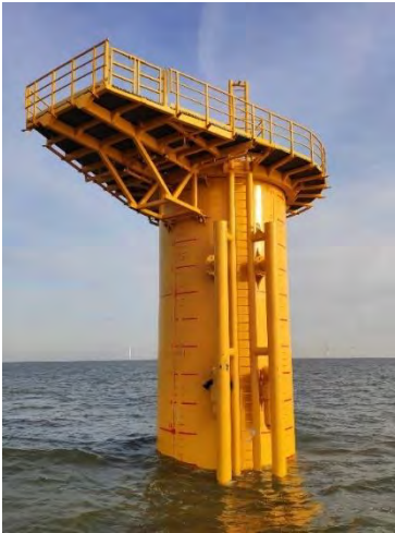
Figure 4-18: Exemplary installed monopile with transition piece [73]
