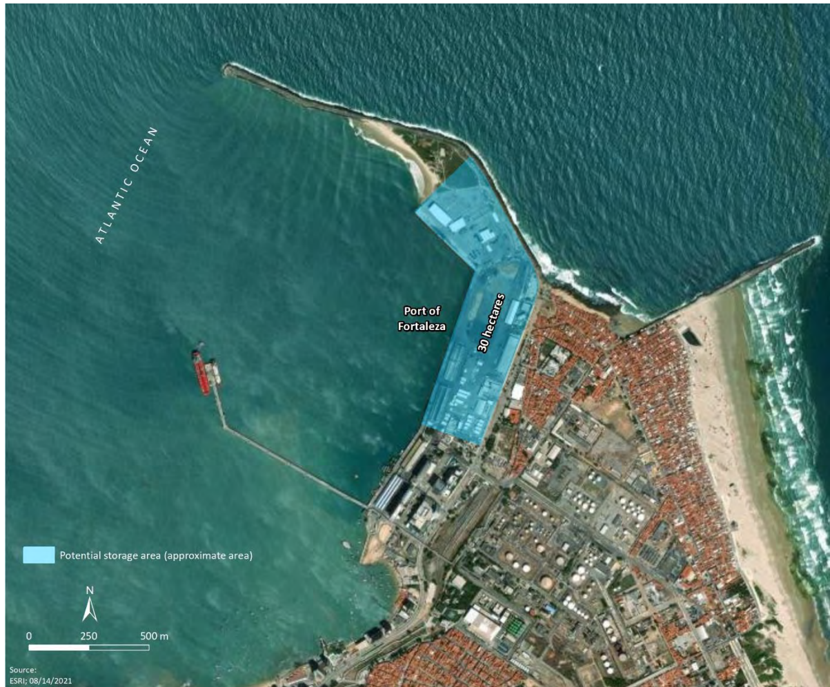
Figure 6-4: Aerial view - Port of Fortaleza
