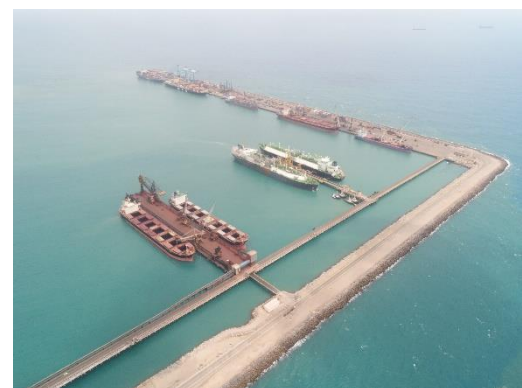
Figure 6-14: Pecém bridge and breakwater, photo courtesy of port of Pecém
