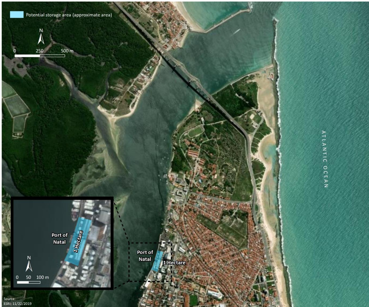
Figure 6-5: Aerial view - Port of Natal
