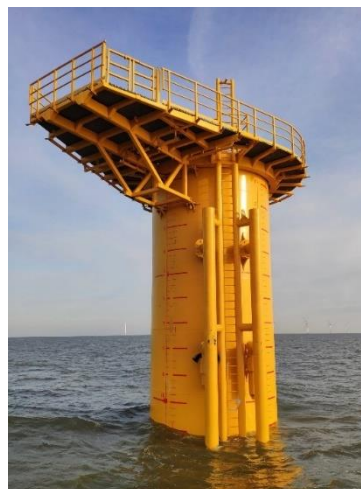
Figure 4-18: Exemplary installed monopile with transition piece [73]
