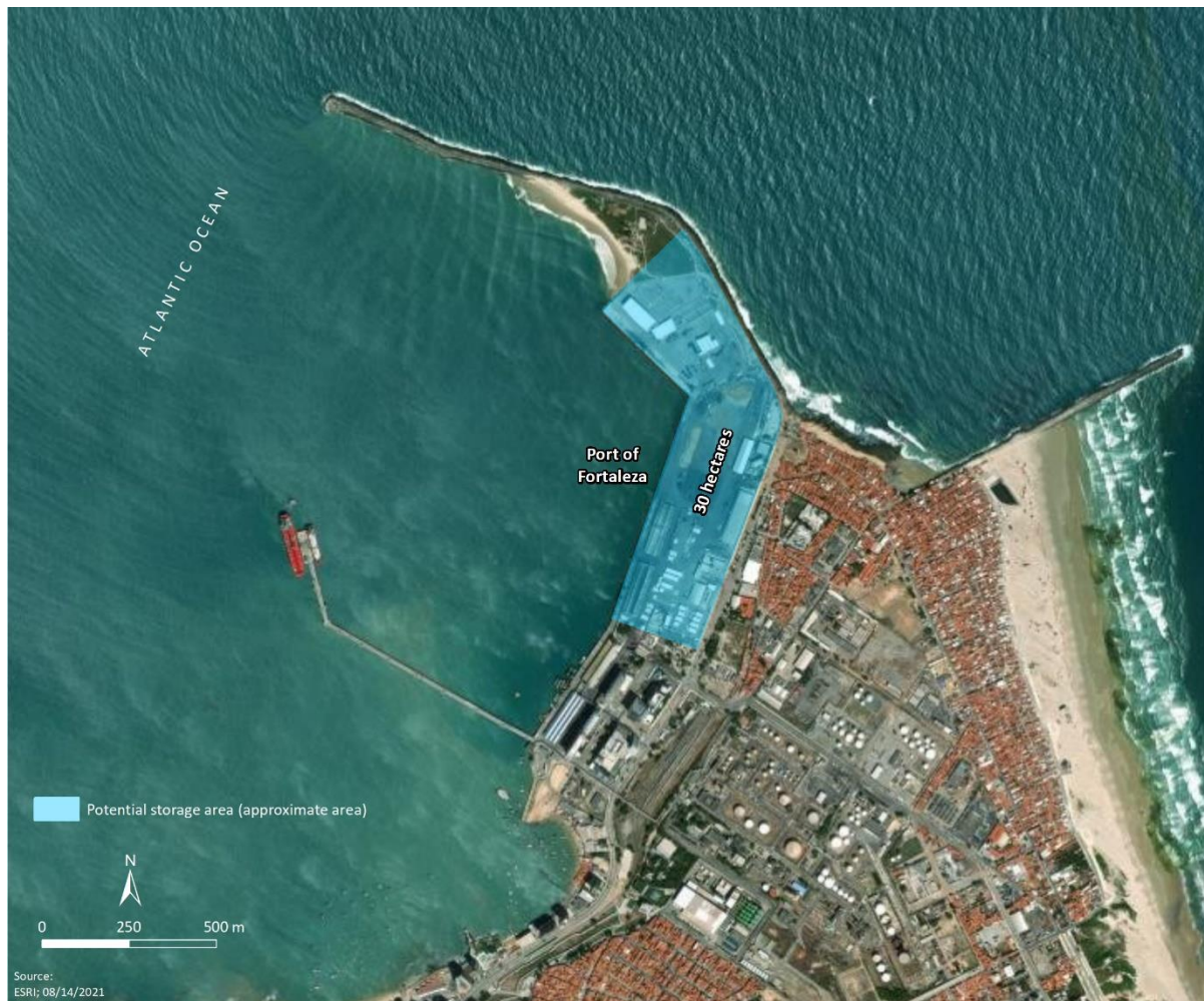
Figure 6-4: Aerial view - Port of Fortaleza
