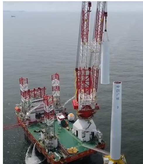
Figure 6-12: WTG assembly offshore [64]
