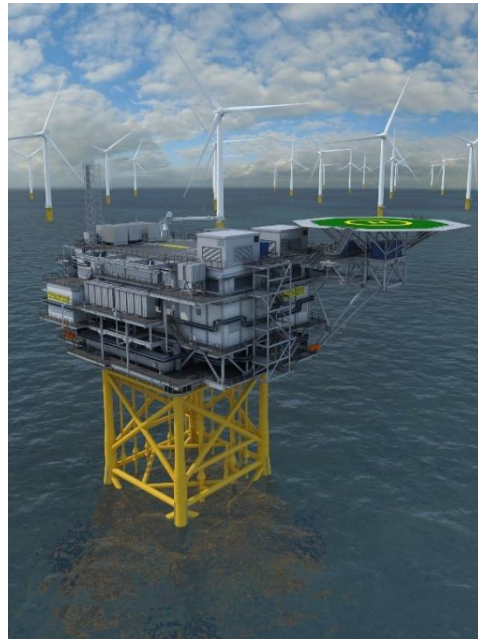
Figure 4-13: Offshore substation rendering of topside and jacket [73]
