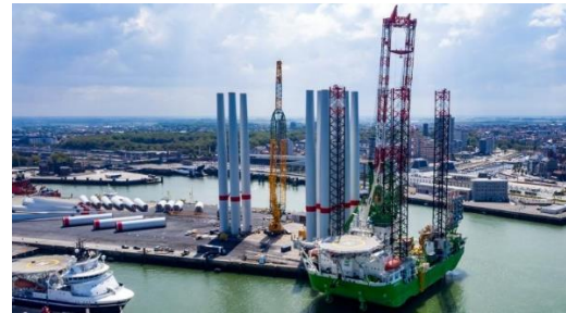
Figure 6-17: WTG pre-assembly at quayside [65]
