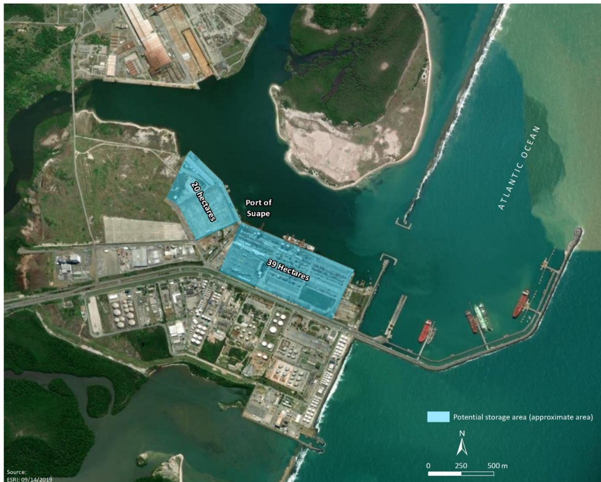
Figure 6-6: Aerial view - Port of Suape
